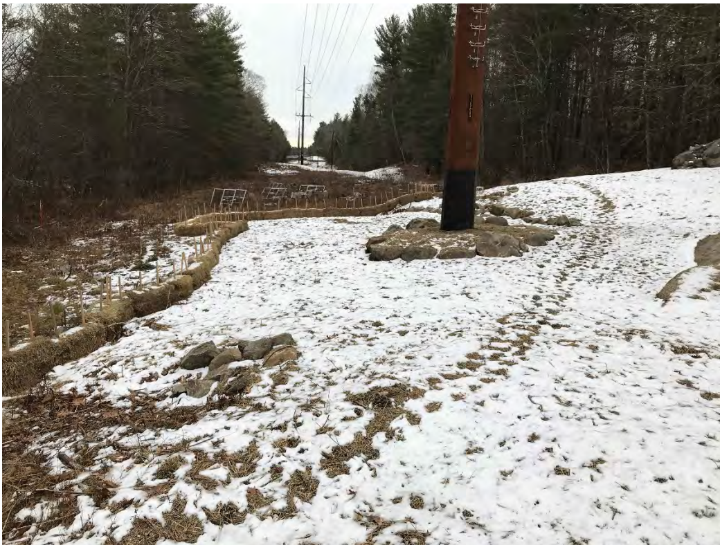
Fig 6: Str. 89 work area. Viewing southeast. (01-11-21)
