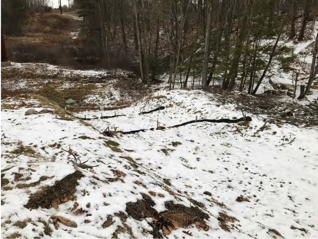
Fig 9: Lower portion of slope between Strs. 28 and 29. Viewing northeast. (01-11-21)
