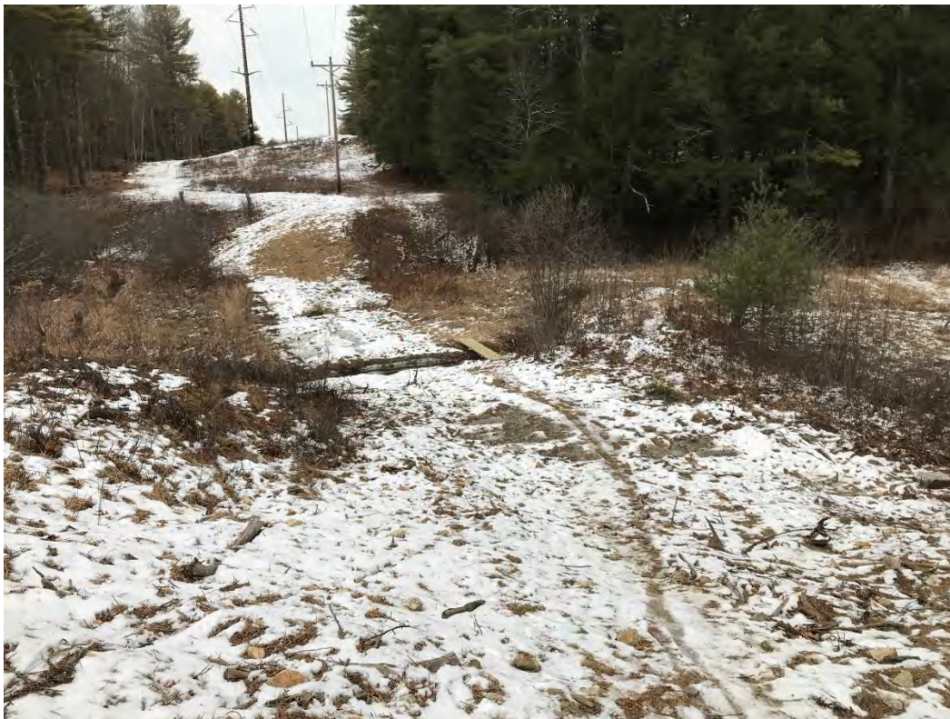
Fig 8: Stream DS46 between Strs. 51 and 52. Viewing northeast. (01-11-21)
