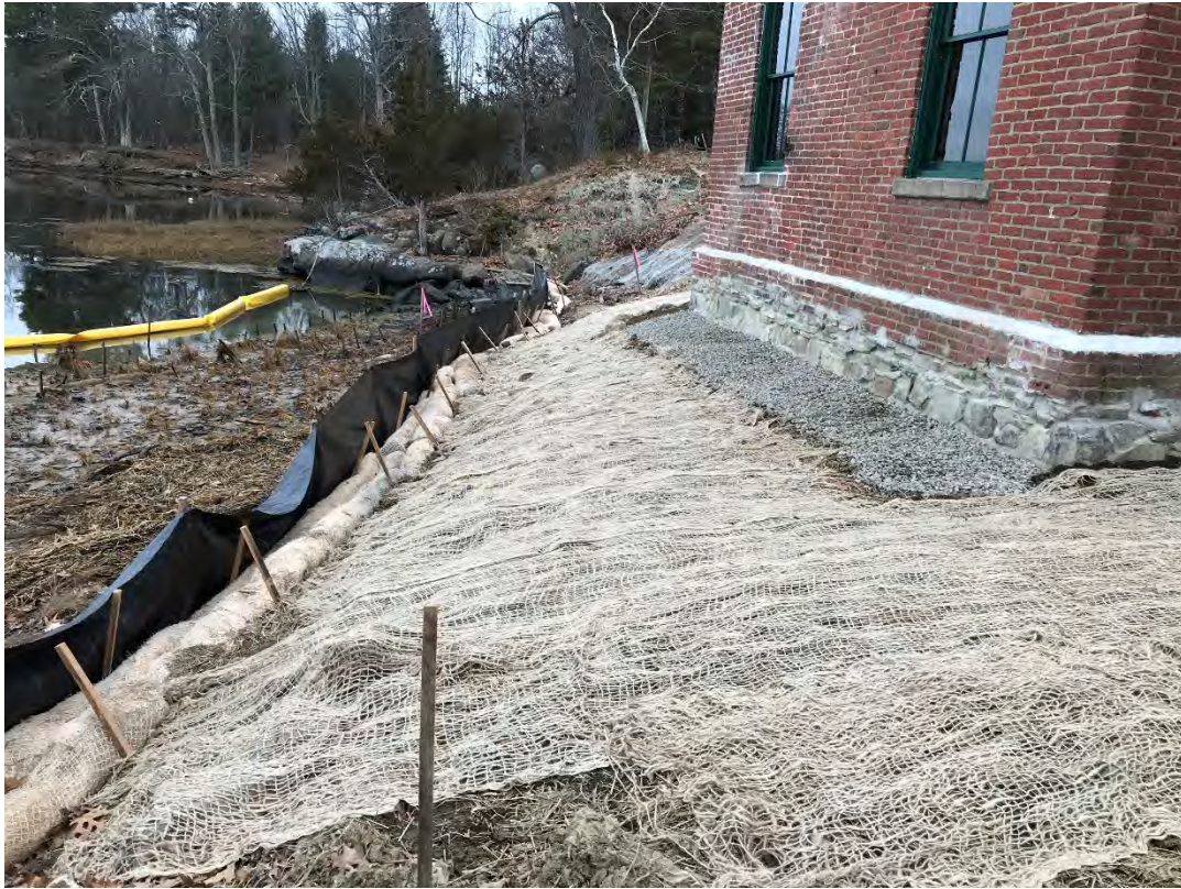
Fig 3: Stabilized slope between the cable house and salt marsh restoration at the Eversource property/west side of the bay. Viewing south. (01-11-21)
