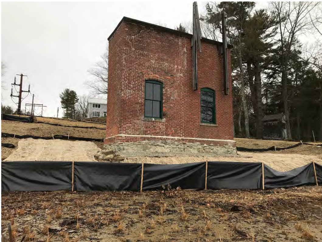
Fig 4: Stabilized slope around the cable house at the Eversource property/west side of the bay. Viewing west. (01-11-21)
