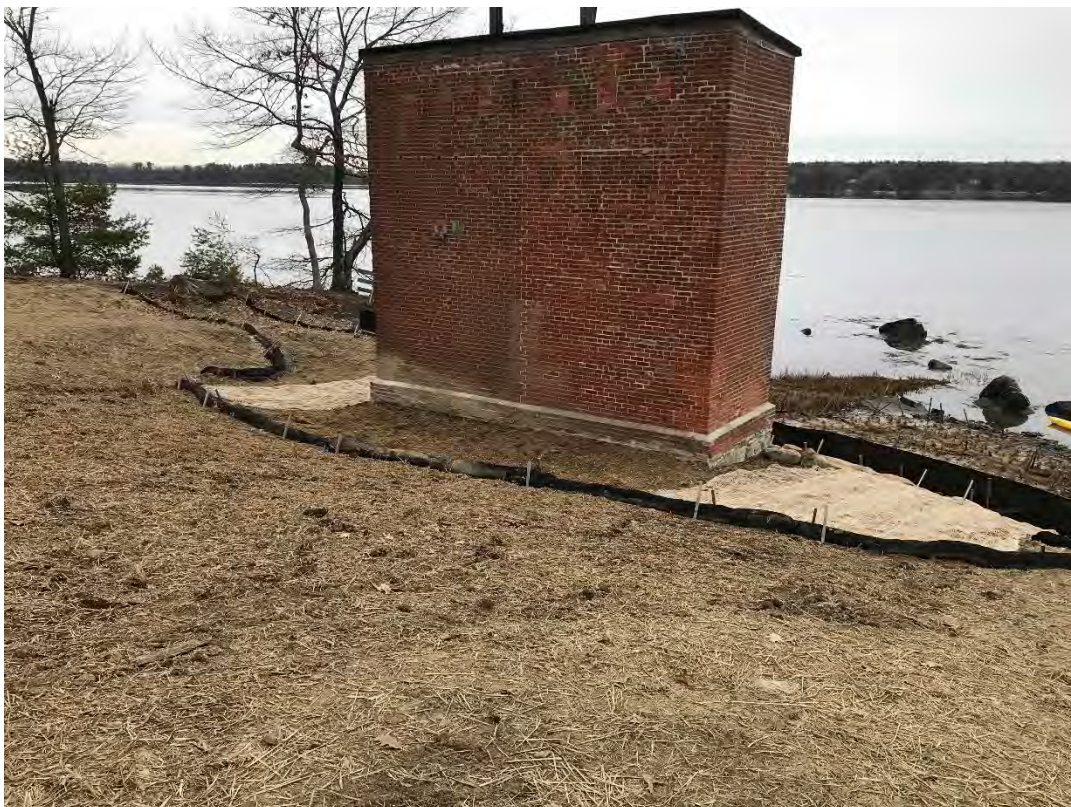
Fig 2: Slope leading down to cable house and salt marsh restoration at the Eversource property/west side of the bay. Viewing northeast. (01-11-21)
