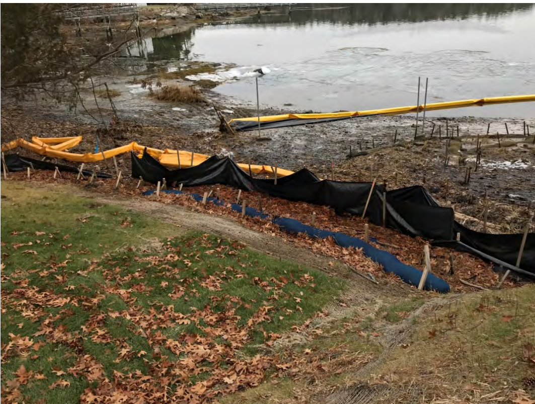
Fig 12: Toe of the slope at Gundalow Landing/east side of the bay. Viewing south. (01-11-21)
